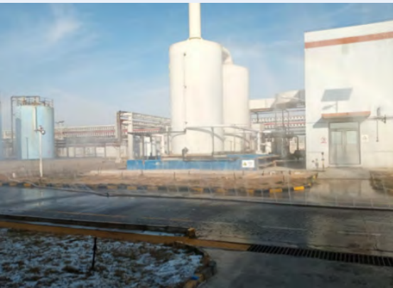
Toxic Gas Suppression with Water Mist
