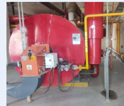
Natural Gas Upgrade for Thermal Oil Heaters
